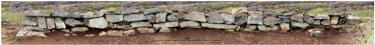
Figure 7: The east facing of wall build (13639).
