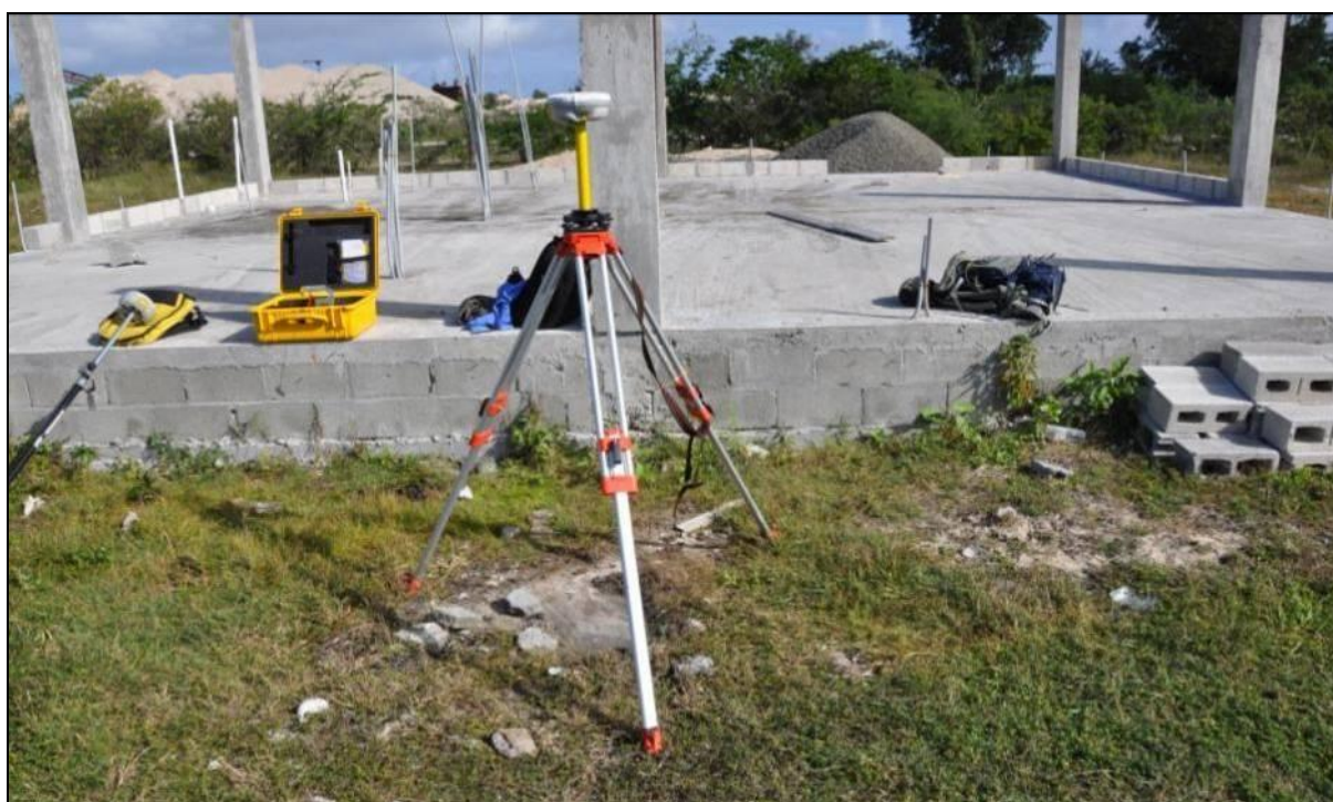
Figure 17. The base station at River. Looking N. (Photo FSI.)
