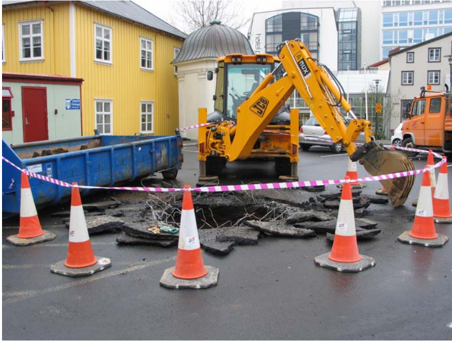
Figure 2. Excavation of trench [1]; 2 nd May 2007.
