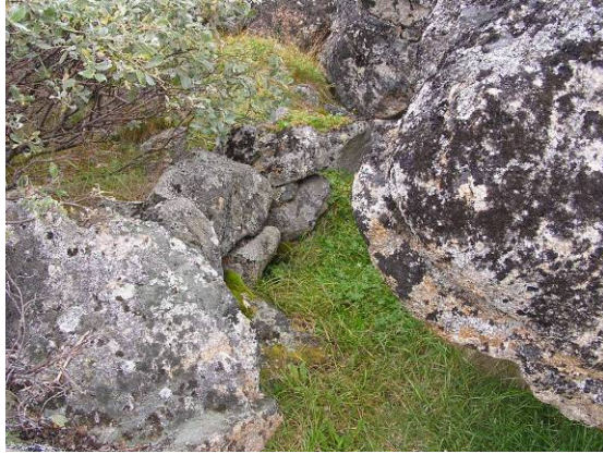
Close-up of the wall under boulder B, looking north.
