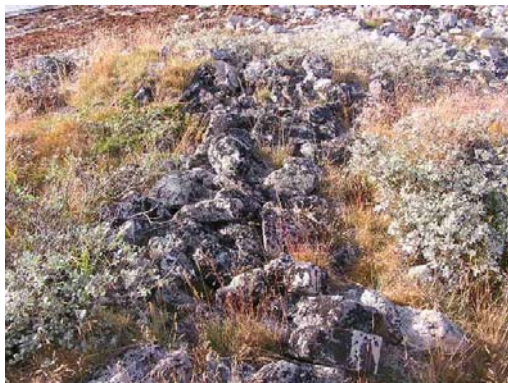
Detail of collapsed wall on the farm mound, looking north.
