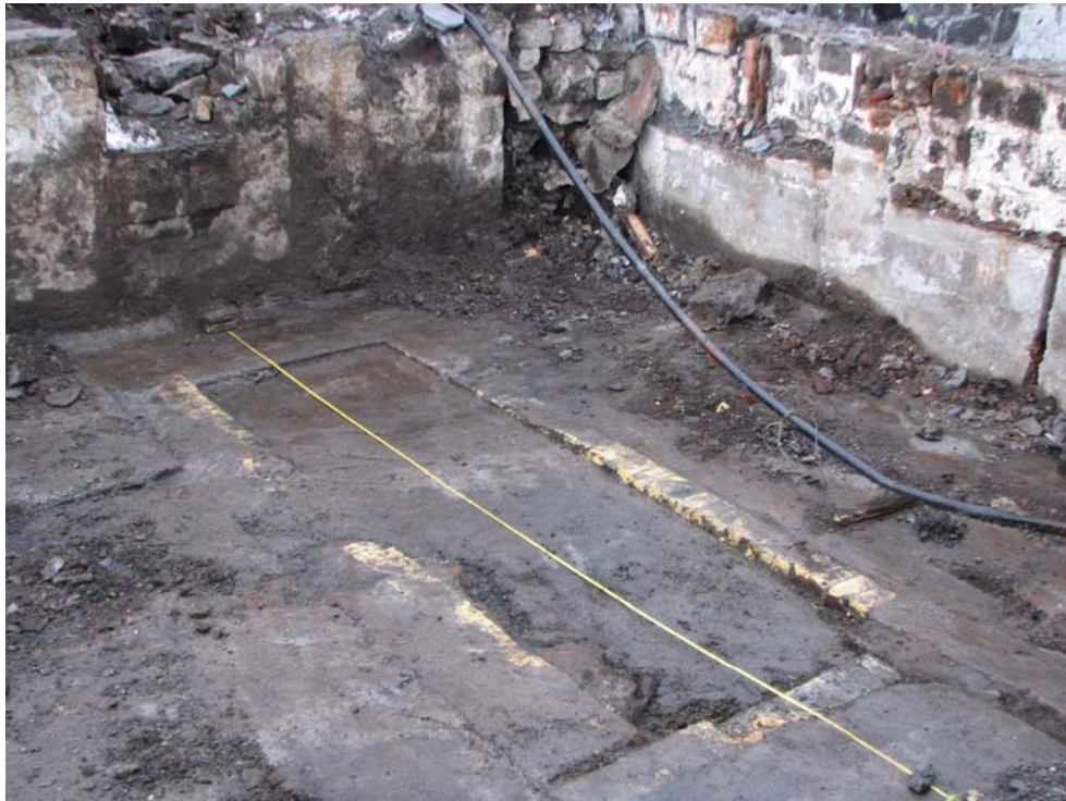
Figure 12. Brick feature in base of [105]. Looking south west. Wall in background is part of [70] for building [45] and where objects were found on its ledge.
