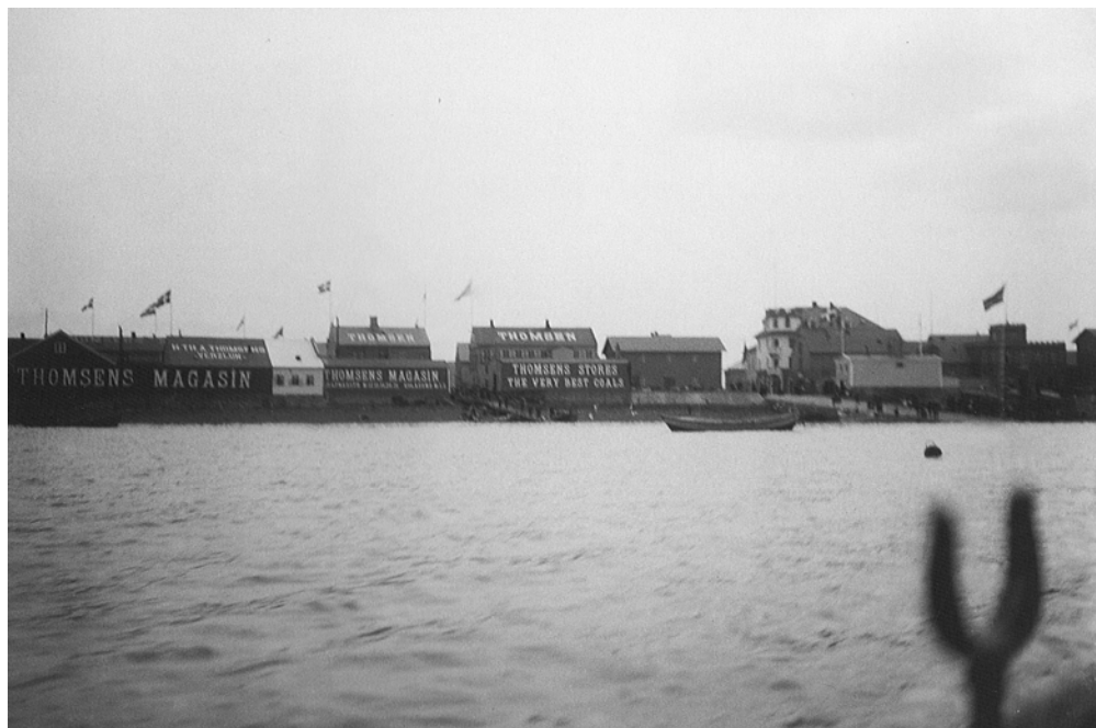
Figure 40. The water front in c. 1909 from a boat looking south (Friis No 47).
