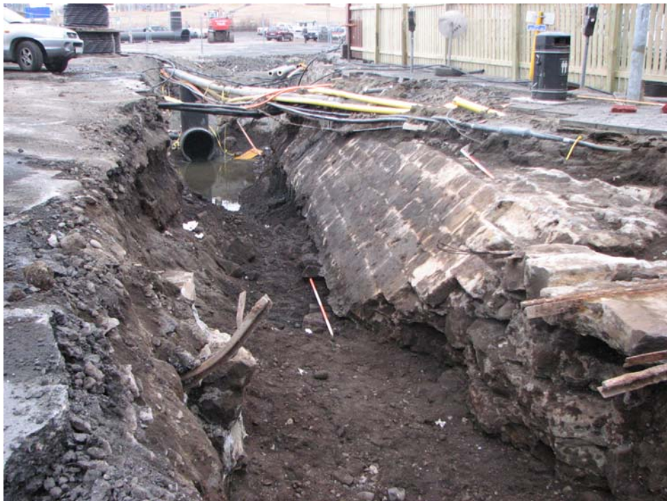
Figure 25. The water front [175] in area 5 with iron tracks (2m scale). Looking east.
