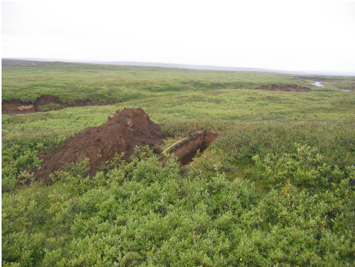
Fig. 33. Trench 1 from the south.
