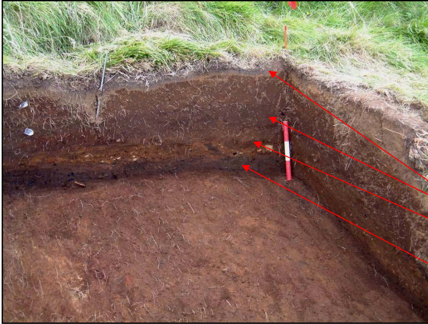
Fig. 12. NW corner (uphill) of the Unit K at the level of context 07. Note the thick modern turf and the broad band of mixed infill (03) below.
