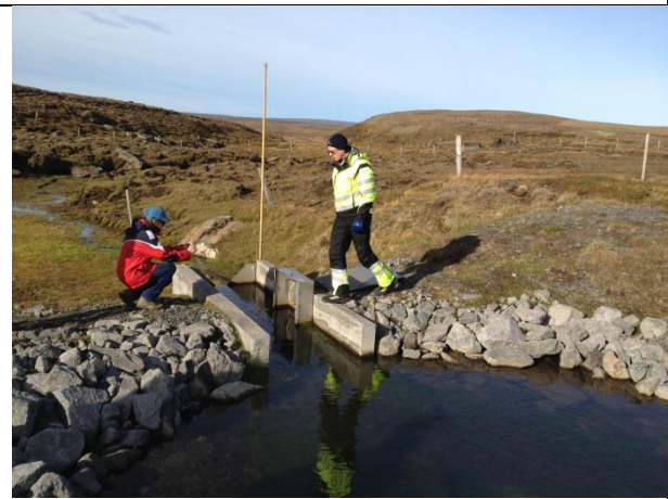
Photo 34: Kolka dam seepage monitoring
