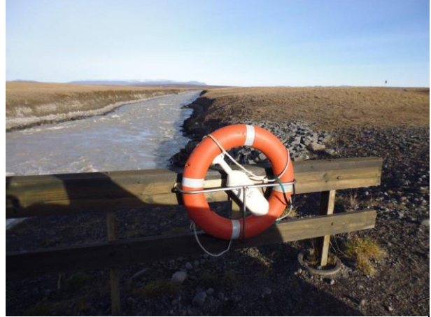
Photo 10: Public safety measures - rescue equipment on bridge over waterway
