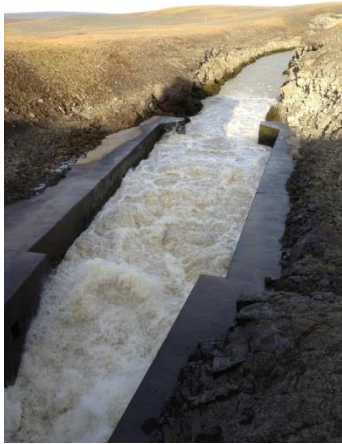
Photo 9: Kolka dam outlet
