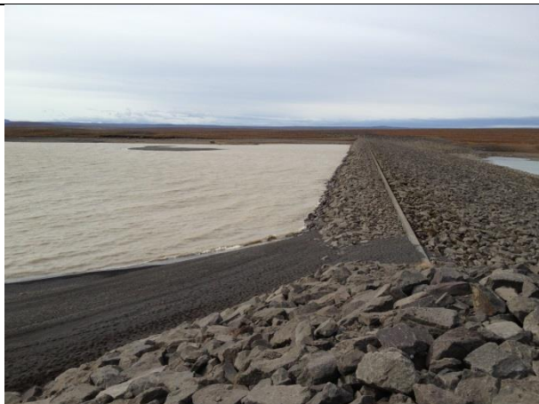
Photo 5: Blanda dam spillway (600 m 3 /s capacity)
