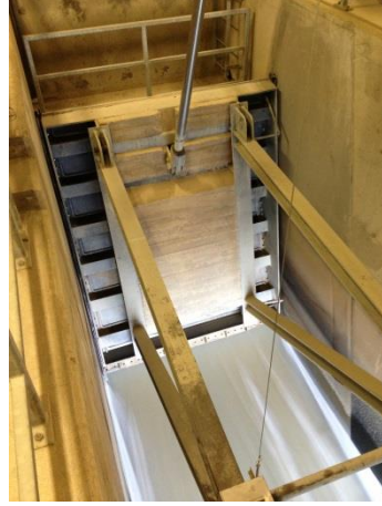
Photo 8: Kolka dam gate
