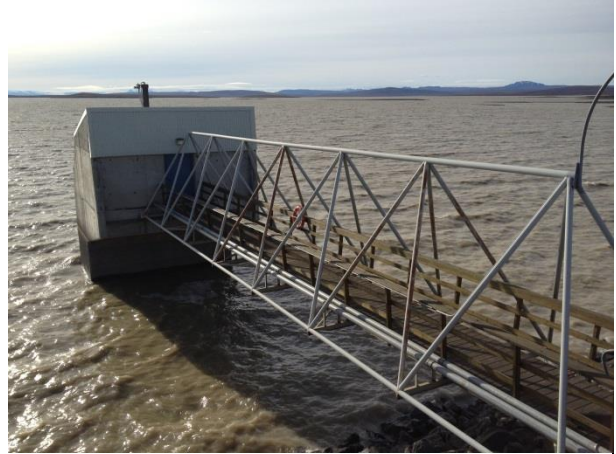
Photo 4: Blanda dam bottom outlet gate house
