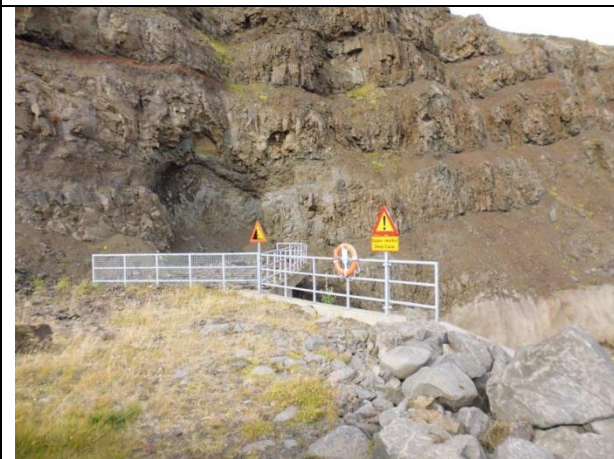
Photo 35: Public safety measures - Blanda tailrace
