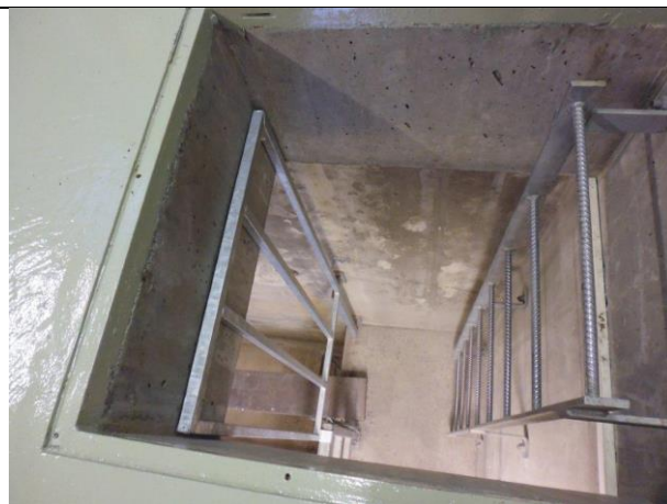
Photo 38: Safety measures – barrier behind ladder
