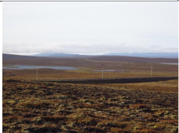
Photo 30: Power distribution lines along road upstream power station
