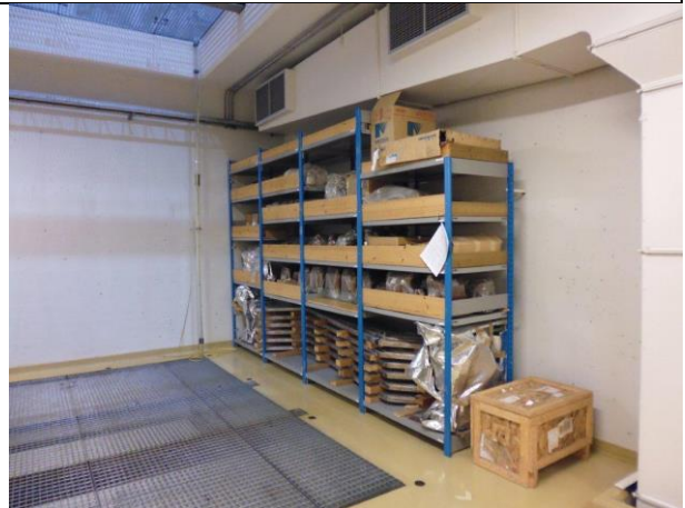
Photo 28: Blanda power station housekeeping - spare parts storage
