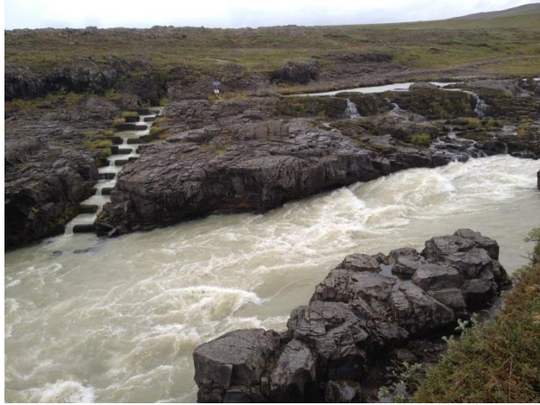
Photo 19: Fish ladder on Blanda River 2 km upstream from mouth (improved by project)
