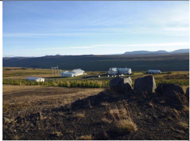
Photo 26: Blanda power station
