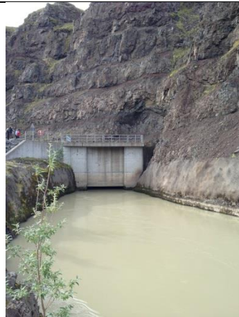
Photo 12: End of powerhouse tailrace tunnel
