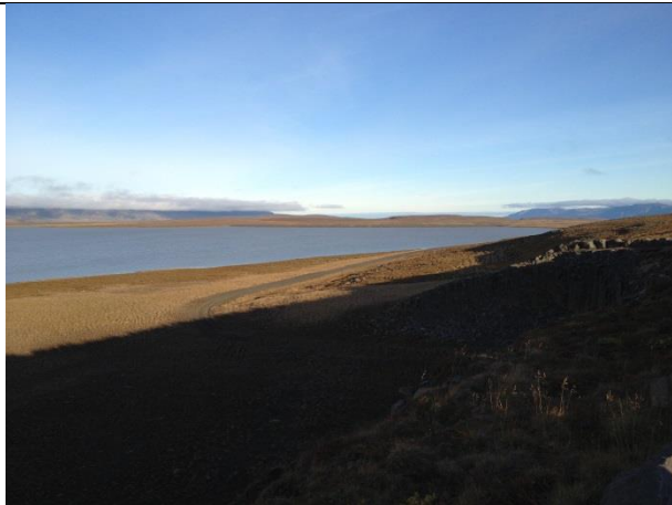
Photo 11: Gilsarlón intake reservoir (5 km 2 )
