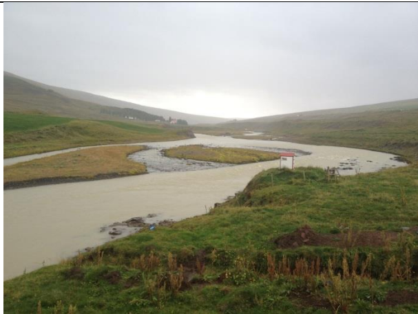
Photo 15: Langamýri gauging station 6 k downstream of tailrace; note overgrown gravel banks due to reduced flooding
