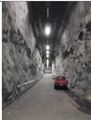
Photo 41: Blanda power station access tunnel with emergency lighting
