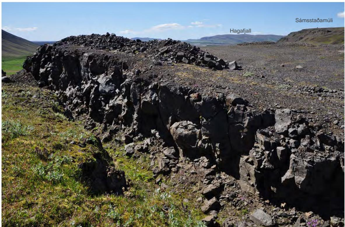
Figure 7-5 Picture taken close to the end of the planned headrace canal at about station 0+530 with the trench in the figure being where the left bank will be. The cut rock in the trench is probably the same as the 5 m thick uppermost tholeiite basalt seen in BF-19 at elevation 239 m a.s.l. to 243 m a.s.l. Viewing west-southwest. Photo: Snorri P. Snorrason 10 July 2012.
