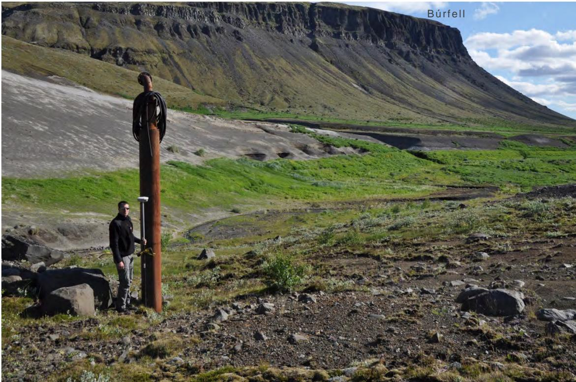
Figure 7-11 Close-up of well BD-1 that was drilled for pumping test in 1984. As can be seen from the height of the surveyor and the exposed casing the excavation at the place is 3-4 metres. Viewing south with mountain Búrfell in the background. Photo: Snorri P. Snorrason 10 July 2012.
