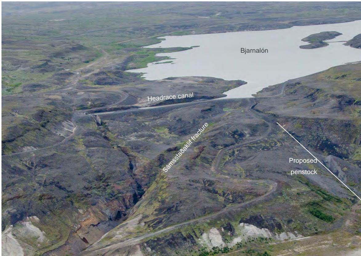
Figure 7-1 Sámstaðaklif-fracture meeting the headrace-canal and diversion dike of Búrfell Station in the centre-right. Location of penstock for Búrfell Extension. Photo: Emil Þór Sigurðsson 16 August 2012.
