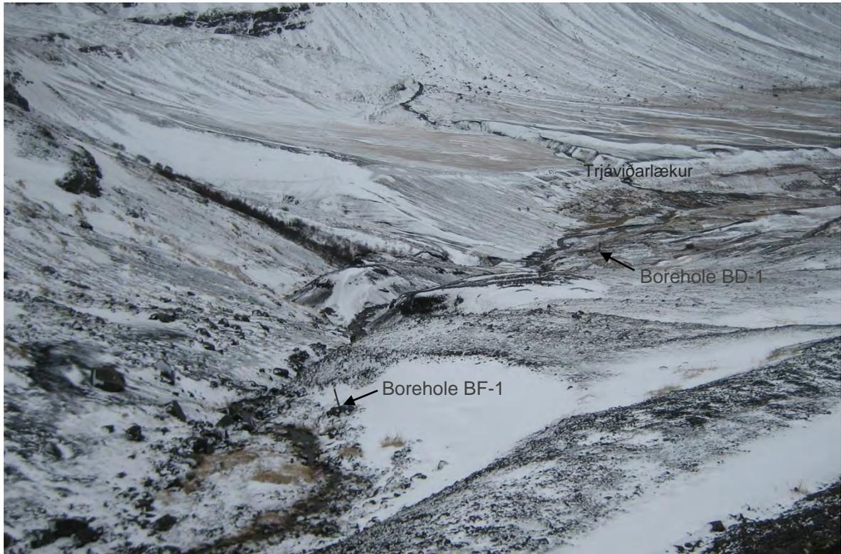
Figure 7-4 Viewing south-southwest with cored borehole BF-1 from 1980 in the foreground and pumping well BD-1 from 1984 at proposed surface powerstation lot. Trjáviðarlækur and other streams opening out to the tailrace canal-to-be. Photo: Steinar I. Halldórsson 2 March 2011.
