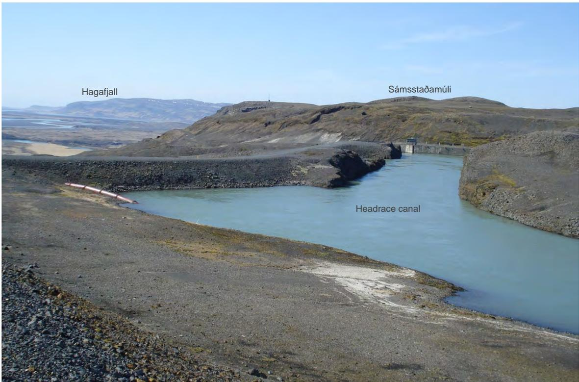
Figure 7-3 Viewing west to Sámsstaðamúli. Headrace canal for the Búrfell Station turning right to the intake. The headrace canal of the Búrfell Extension starts on the nearbank and the pipe in center left passing underneath the diversion dike is located at what will be the right bank of the new headrace canal at about station 0+350. Photo: Steinar I. Halldórsson 3 May 2011.
