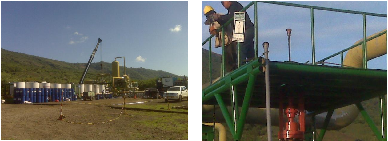
FIGURE 5: Pictures taken during the acid job, November 2009, in well MT42
