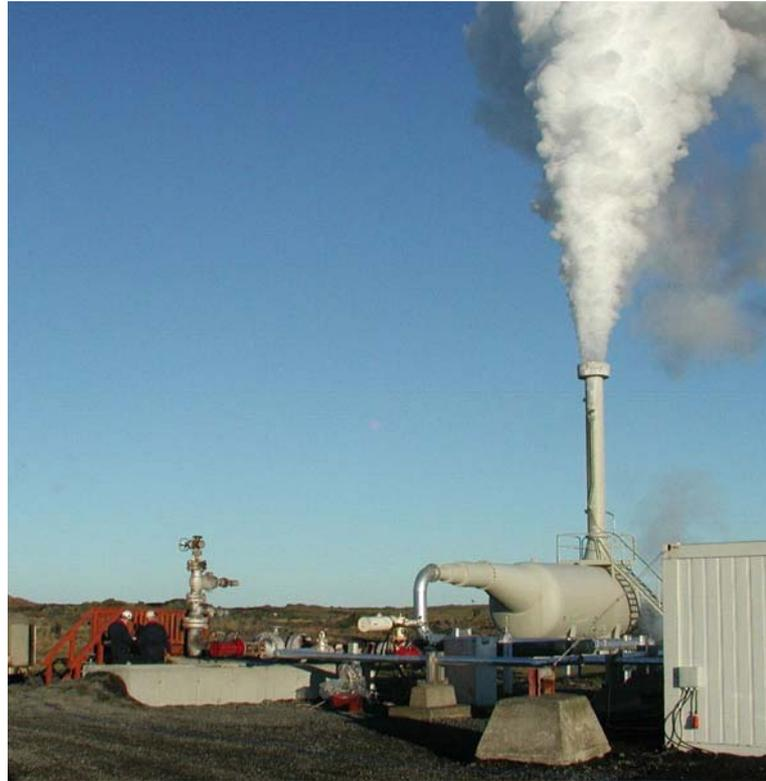
FIGURE 5: Well head, separator and different controlling devices
