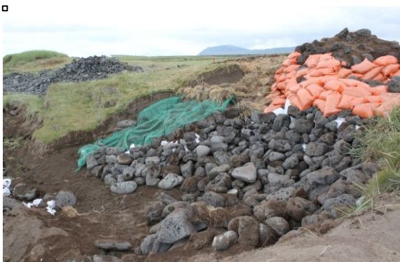
Figure 44 Left. Eroded section covered at the end of season
