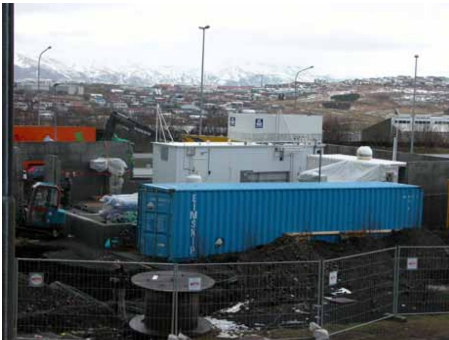
Figure 5 The station on 31 st of March 2003, four weeks before the inauguration.
