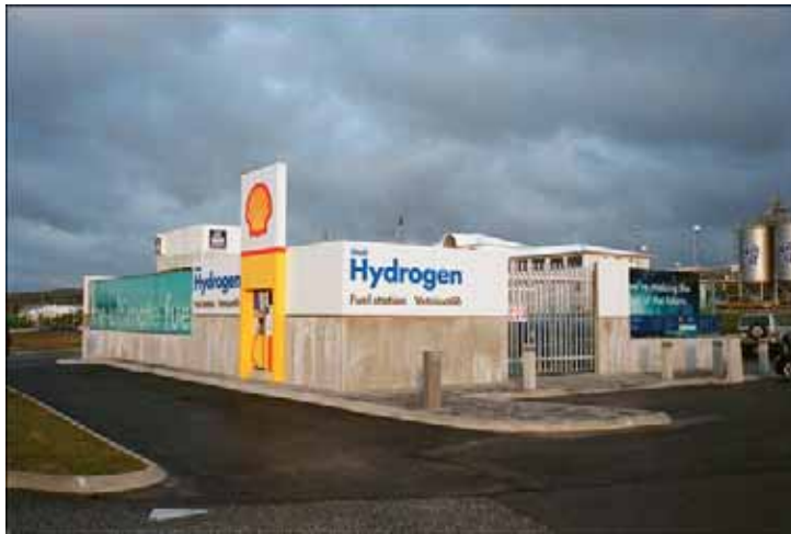
Figure 7 The station seen from the west. The panels in the background to the right carry texts and drawings that explain in Icelandic and English what is hydrogen, how it is made and used in fuel cells
