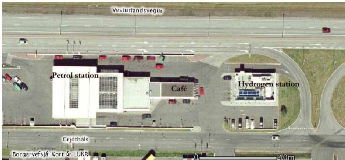
Figure 8 The hydrogen station (to the right) was built beside the main highway that connects the city with all rural areas. It stands aligned with a normal gasoline station (to the left) a coffee and snack bar (in the middle) 15
