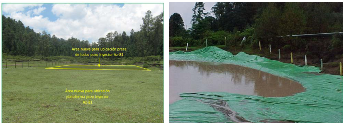
FIGURE 2: Site selected for the mud dam and waterproofed
