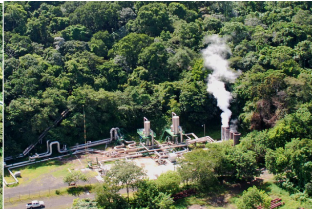
FIGURE 6: Omega bend expansion loop
