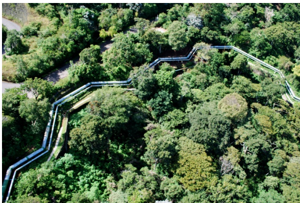
FIGURE 5: V bend expansion loop
