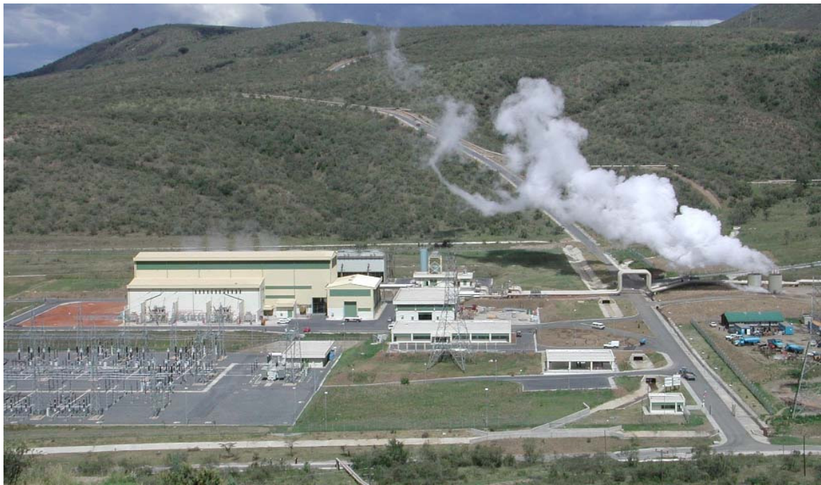
FIGURE 3: Olkaria II power station (105 MW)
