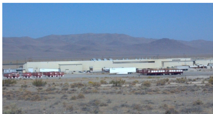
FIGURE 8: Onion dehydration plant
