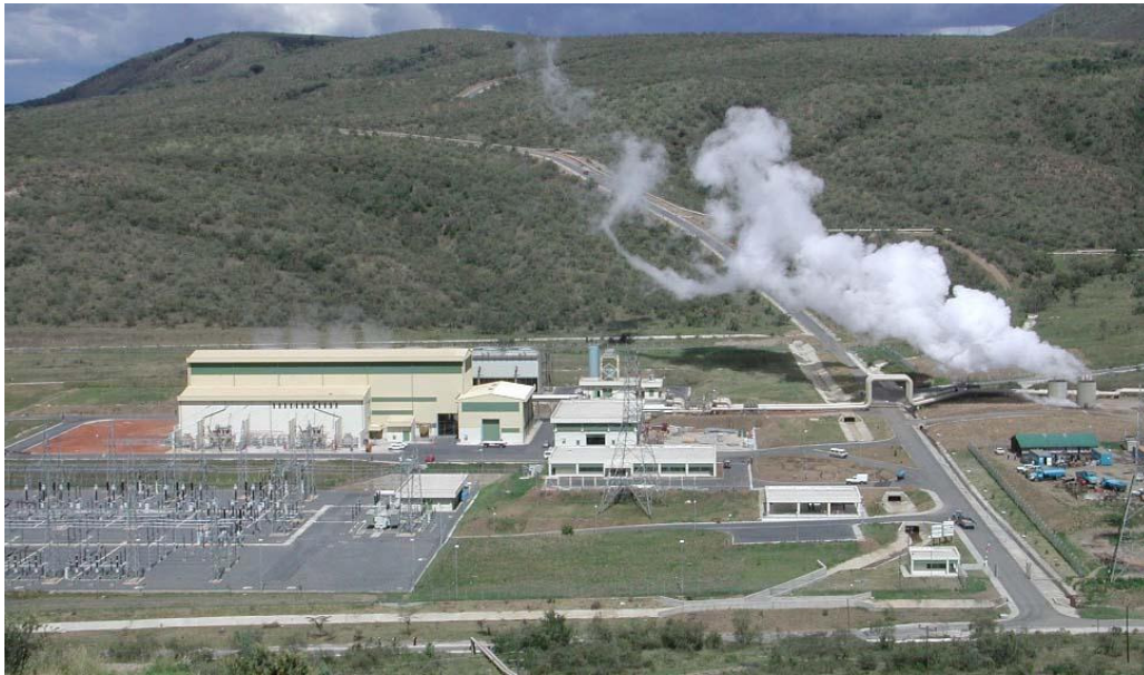
FIGURE 5: Olkaria II power station, commissioned in 2003
