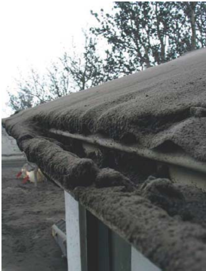
Figure 8. Ash deposited on a tin roof in the area south of Eyjafjallajökul, 16 May 2010. (© Ari Tryggvason.)
