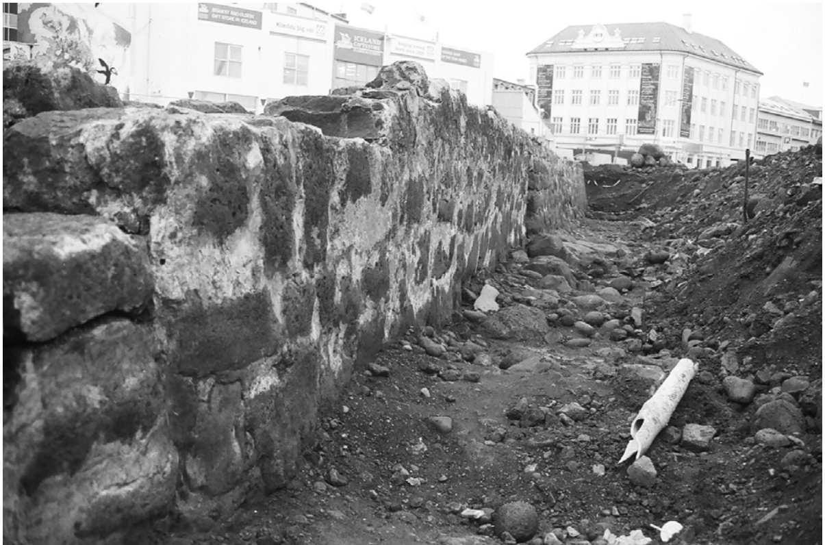
Figure 10. Sea wall looking west. Notice the angle of the wall on the foreground of the picture and its gradual change in angle towards the background.
