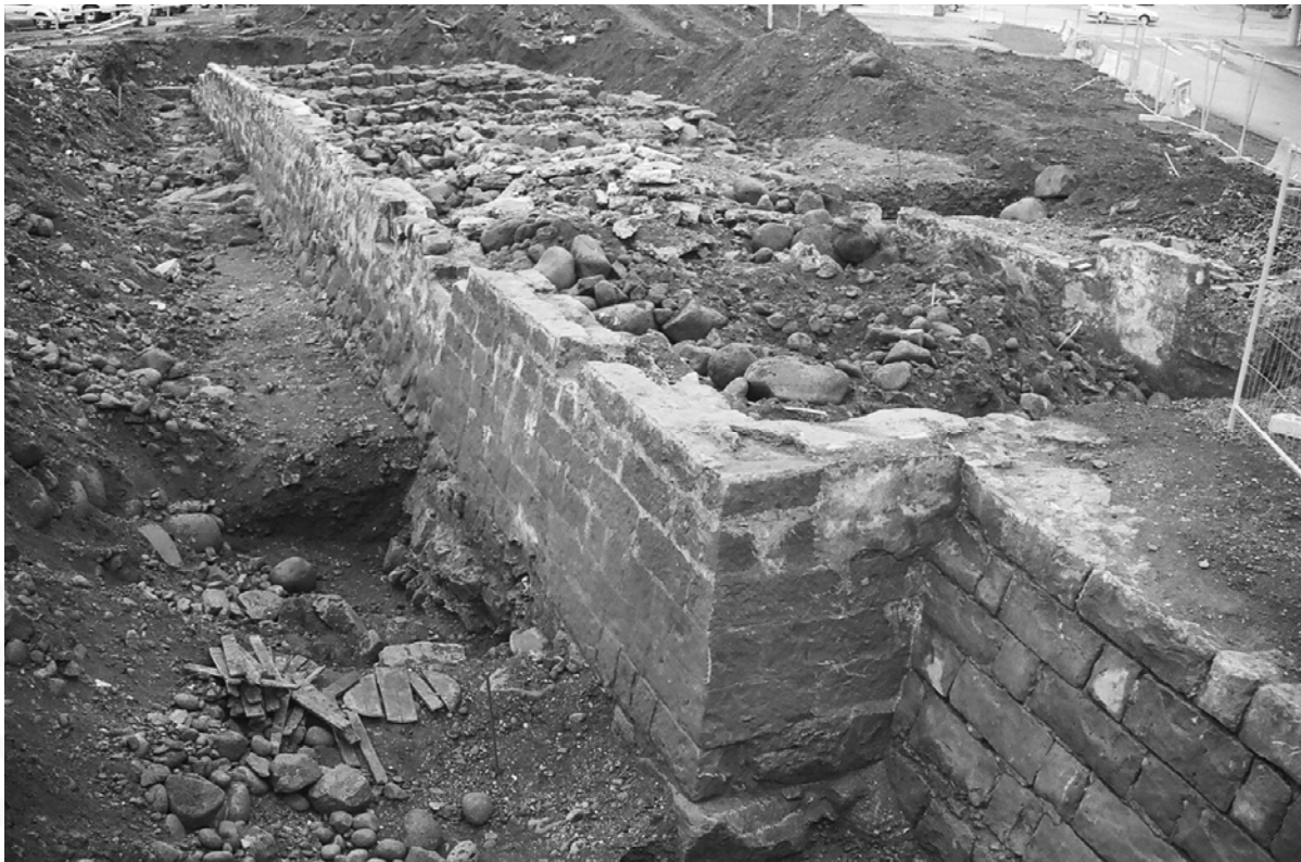
Figure 9. Sea wall, including views across structures (from right to left) [45 (corner of), 200, 274, 275, 276, 327].
