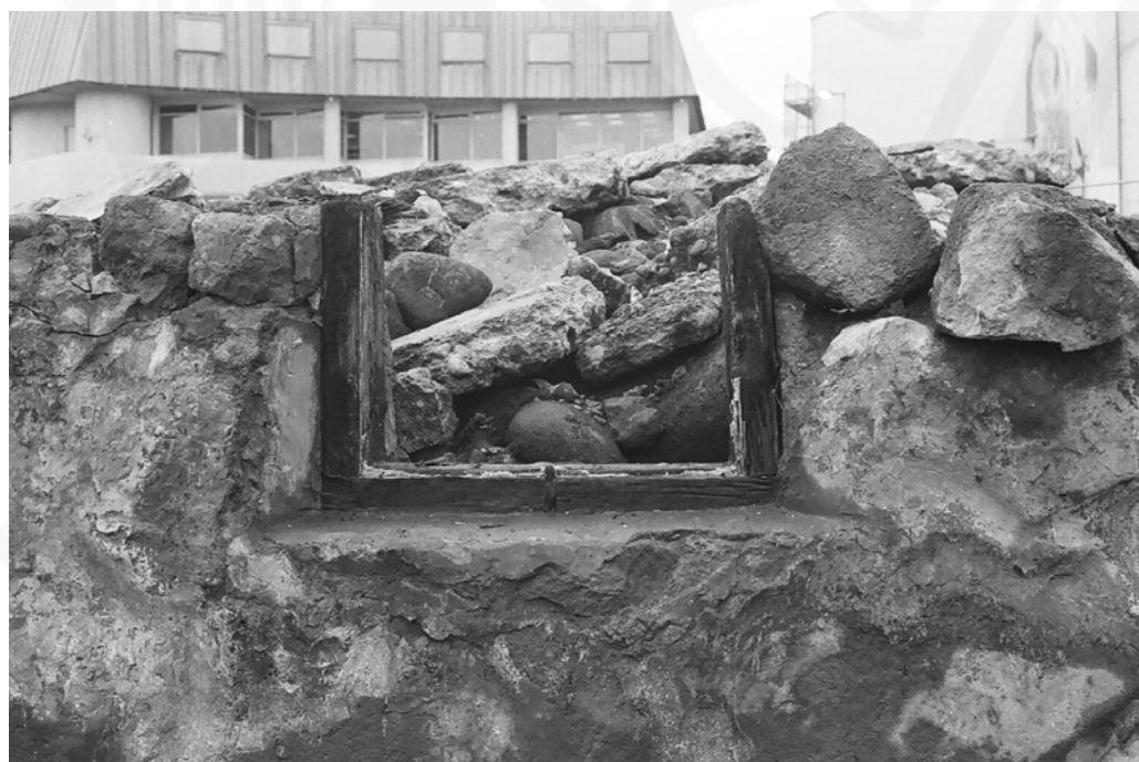
Figure 17. Window in the northern wall of [200]; facing south. The window fronts onto the sea.
