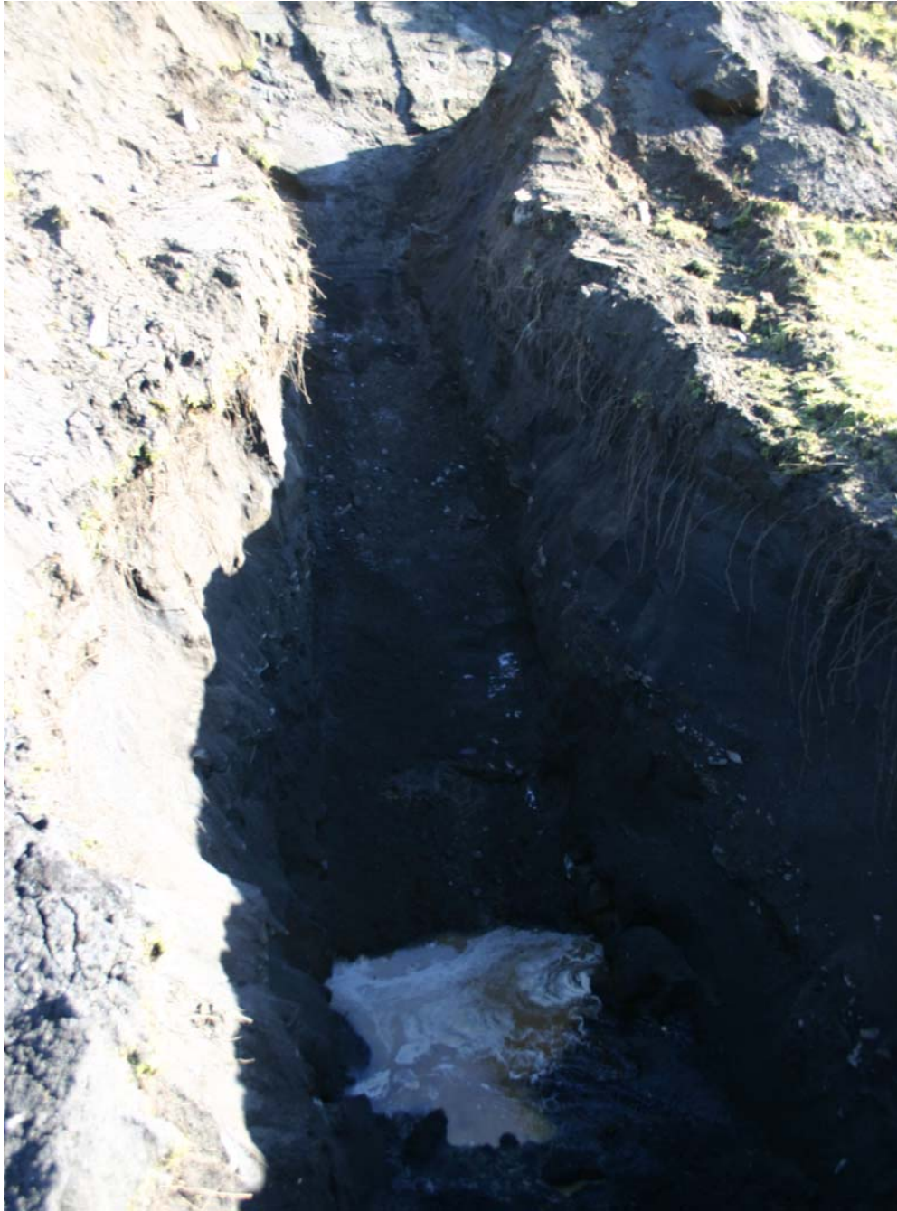
Figure 2-4. Fissure trench AK-1 just after excavation. Unsure signs of a fissure or fault are in the shadow at the light spot just above the inflowing water.
