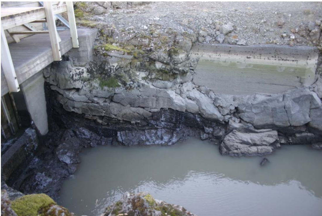
Figure 4-: Leakage from top section of the Þjórsá lava into salmon waterway at Budi waterfall.
