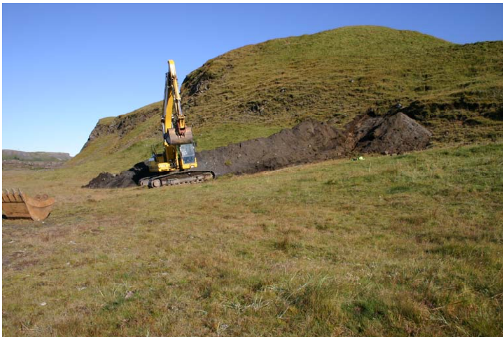
Figure 2-2. Fissure trench AK-1 at Akbraut farm.
