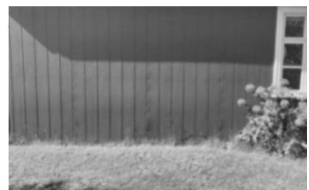
Fig 3. Example of a house, sitting on no foundation. The house sits on top of the soil. Difficult to identify.
