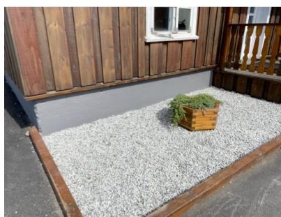
Fig 2. Concrete foundation, the foundation is most commonly hidden and can't be seen. Typical for building built after 1930.
