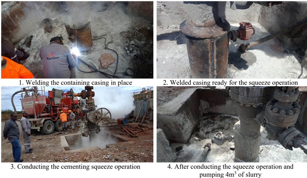
FIGURE 4: Squeeze cementing operation at well OW-740A (KenGen, 2019a)
