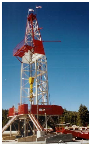
~ 55 m high rotary rig
