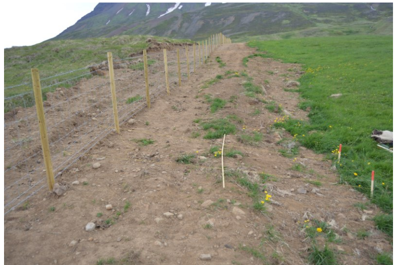
Figure 51: The location of trench 11. On the picture to the right the location of the excavated trench can be seen and the picture to the right shows the location of the trench, before excavation
