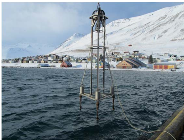
Figure 7. Drilling test at Siglufjordur harbour
