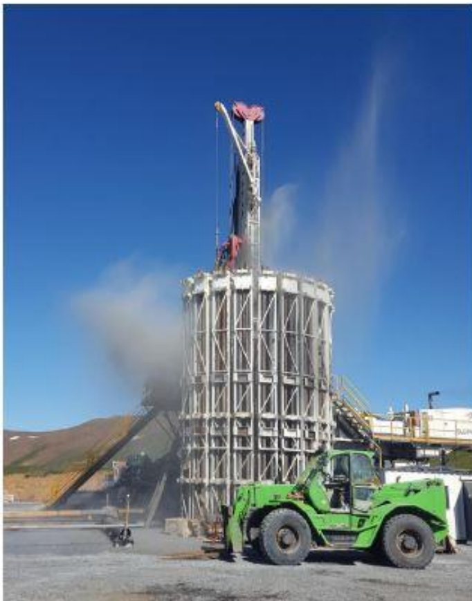
Figure 2. A blow-out from DG-10 at 3:35 pm yesterday.
