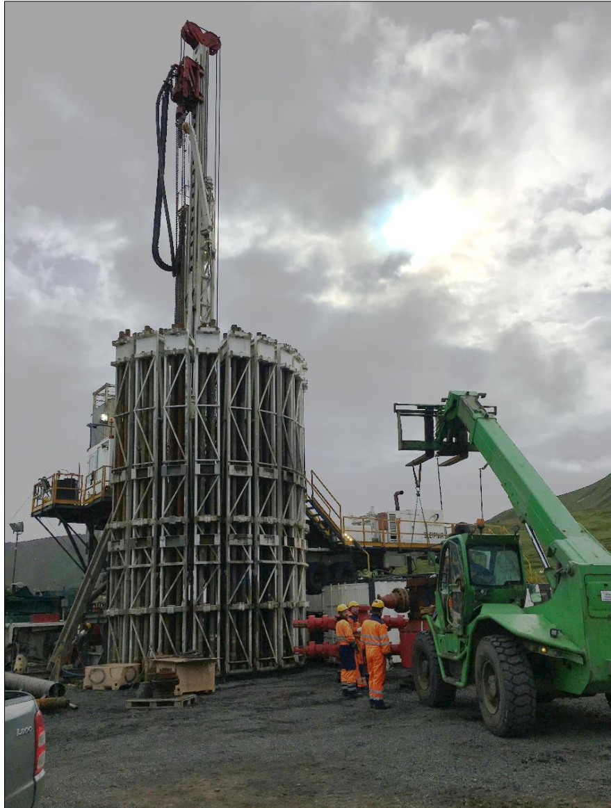
Figure 2. The drill crew at work this morning.
