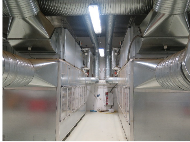
FIGURE 24: Air cleaning room
