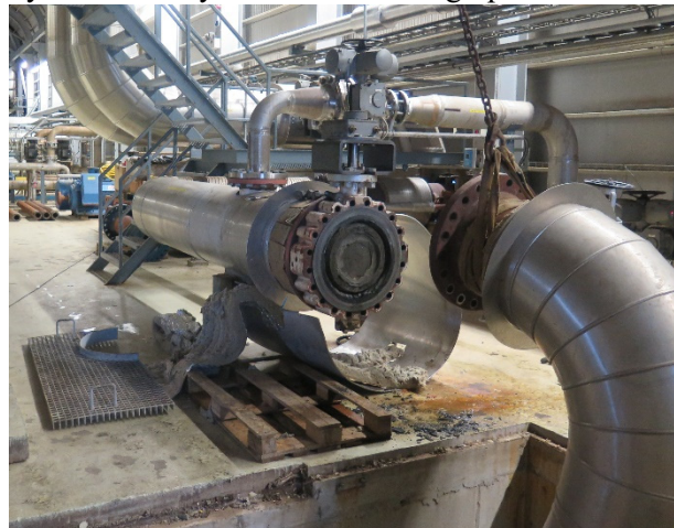
FIGURE 13: Pipeline and valve maintenance
