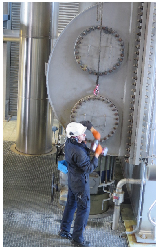
FIGURE 20: Inspection of the condensers
