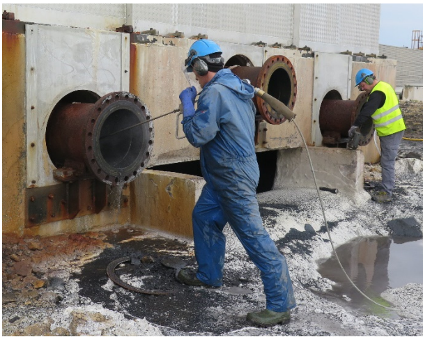
FIGURE 22: Cleaning pipes of silencers by hydro-blast pumps
