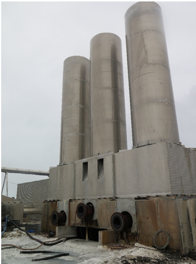
FIGURE 7: Silencers of the power plant
