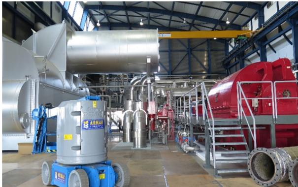
FIGURE 2: Svartsengi power plant
