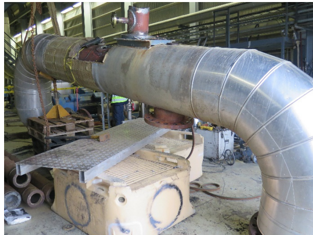
FIGURE 28: Repairing of pipes
