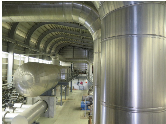
FIGURE 6: Horizontal separators the power plant
