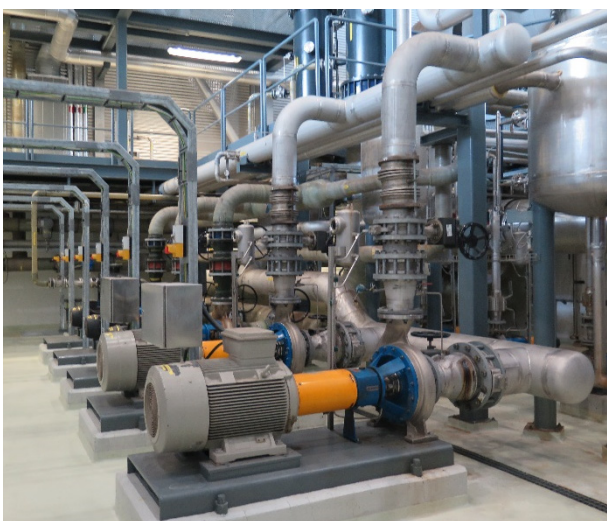
FIGURE 23: Power plant pumps
