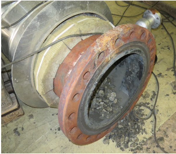
FIGURE 14: Cleaning scaling in pipes
