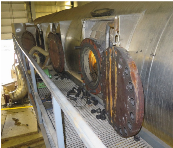
FIGURE 15: Separator inspection during outage
