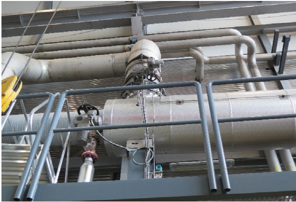
FIGURE 21: Steam ejector
