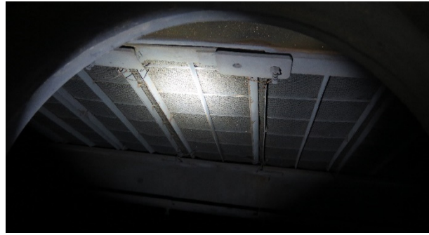
FIGURE 16: Moisture separator inspection during outage
