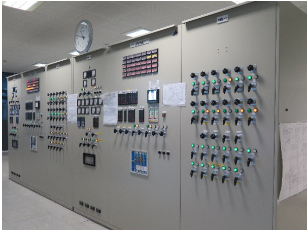
FIGURE 26: Main control room
