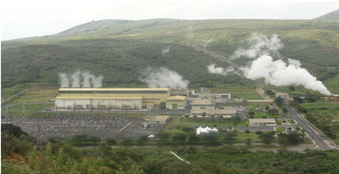
FIGURE 4: A view of Olkaria II power station
