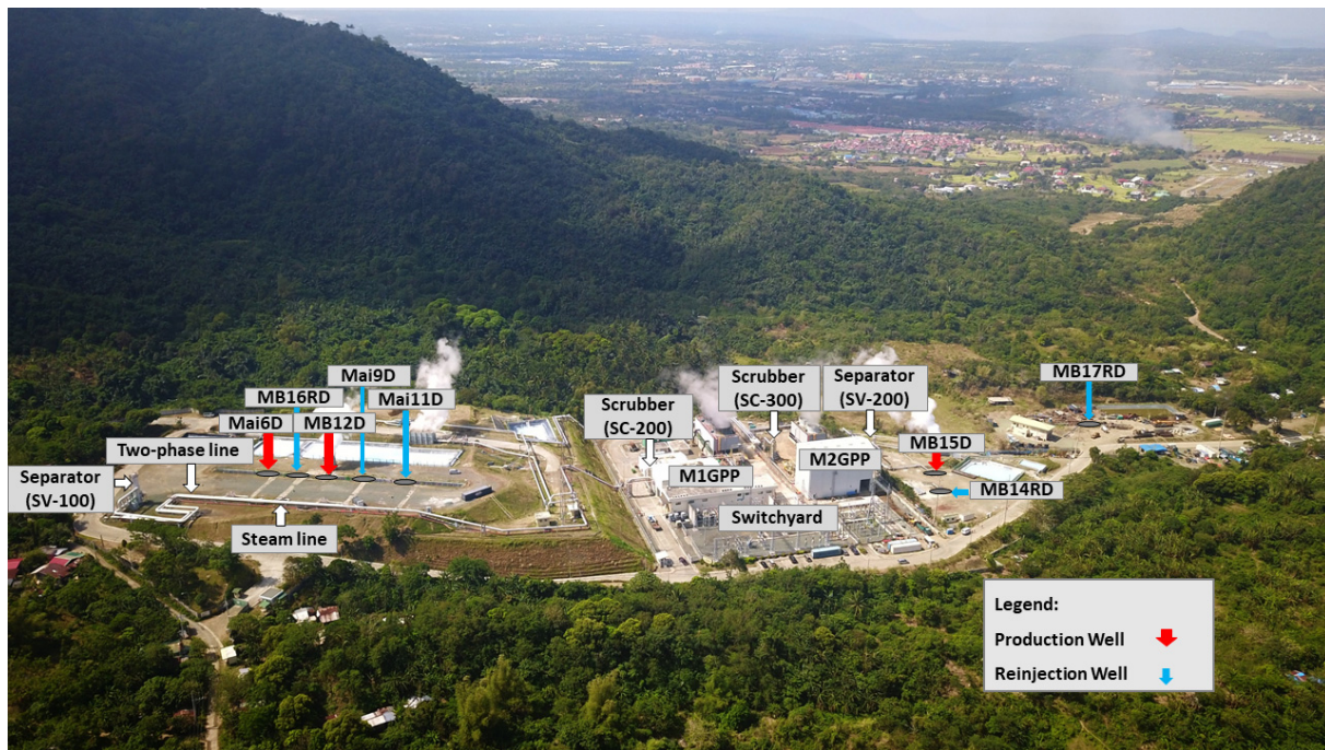
FIGURE 3: Maibarara geothermal field overview
