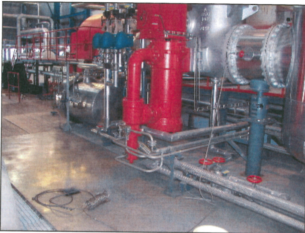
Fig. 1: Steamline after separator but before mist-eliminator
