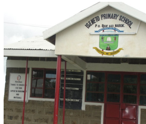
FIGURE 8: Classrooms constructed at Iseneto
