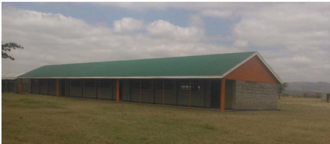
FIGURE 6: New classrooms constructed at Oloirouwa primary school
