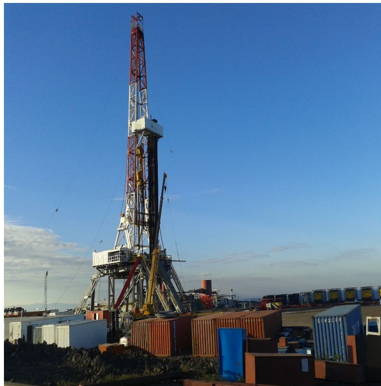
FIGURE 5: Rotary drill rig
