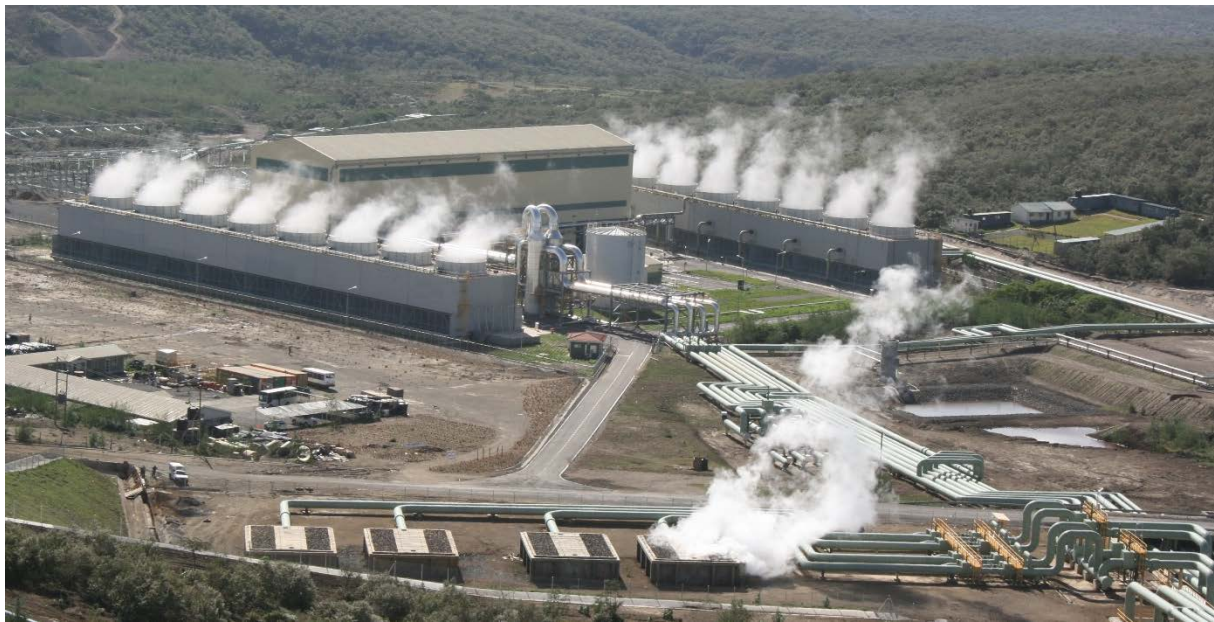
FIGURE 3: The Olkaria IV power station in Kenya, opened in mid-2014, with an installed capacity of 140 MWe from two 70 MWe turbines
