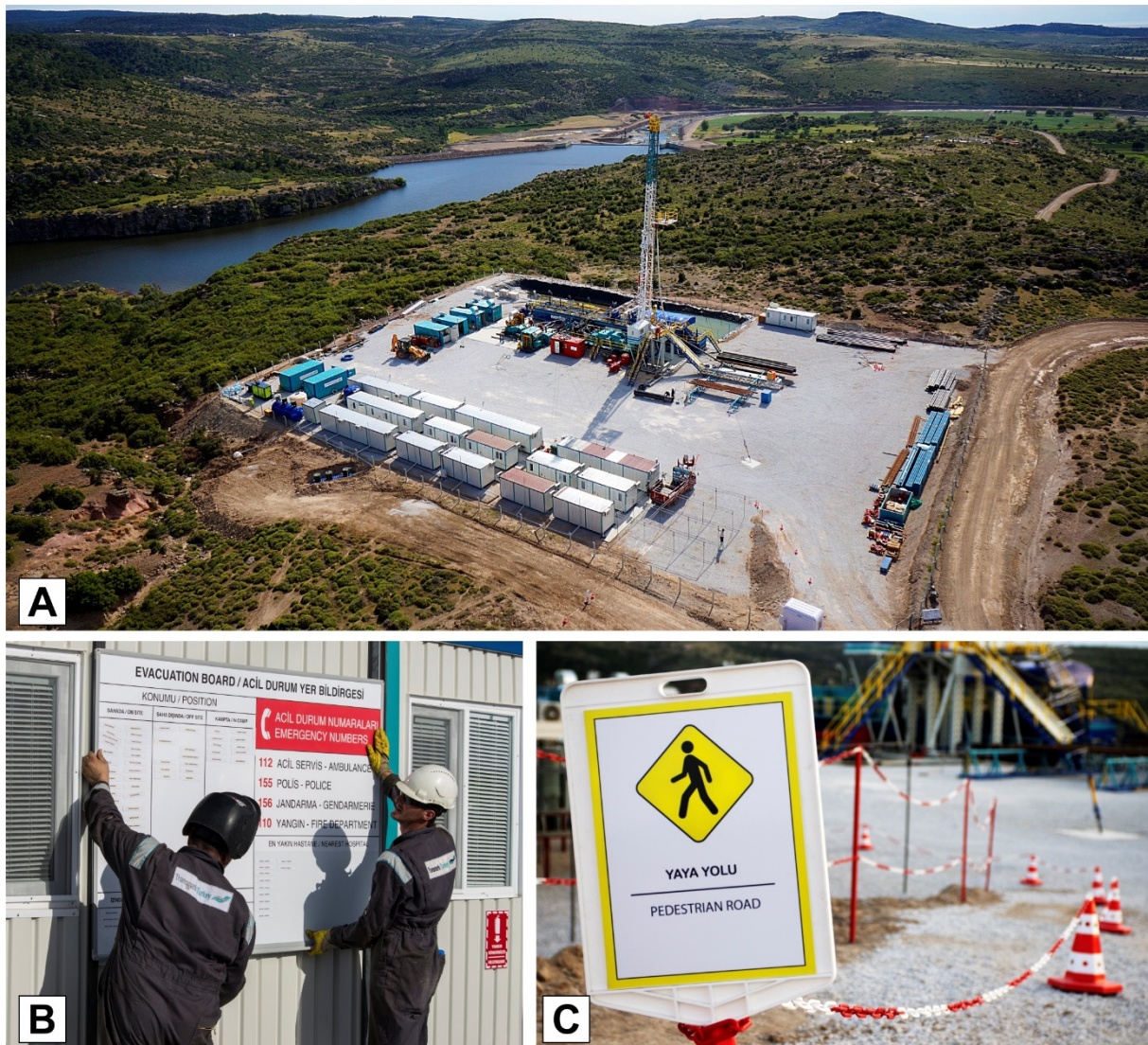
FIGURE 34: Security precautions in a geothermal drilling site; A) Air-view of a typical drilling site; B) Evacuation and warning signs; C) Pedestrian road example (source:Fotokopter-Transmark)
