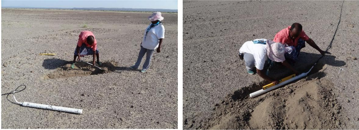
FIGURE 26: Digging of a shallow trench and leveling the magnetic sensor
