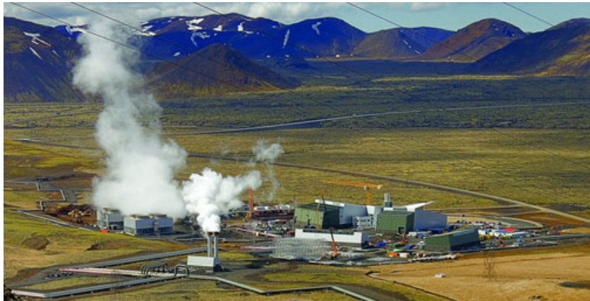
FIGURE 1: Hellisheidi geothermal power plant (Power-Technology.com, 2014)
