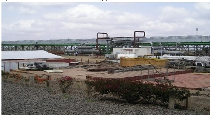
FIGURE 4: Olkaria III 35 MWe power plant under construction
