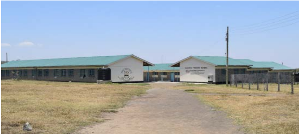
FIGURE 9: A primary school constructed as part of entitlement for the PAPs
