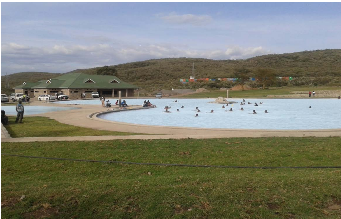
FIGURE 7: A view of the Olkaria Geothermal Spa
