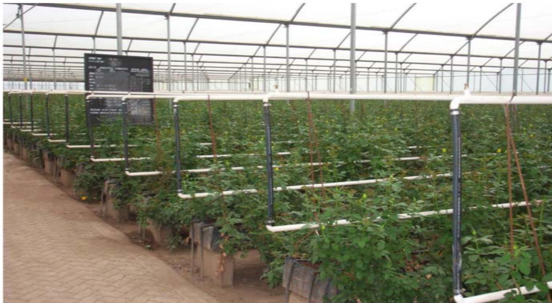
FIGURE 6: Oserian greenhouse heating using geothermal
