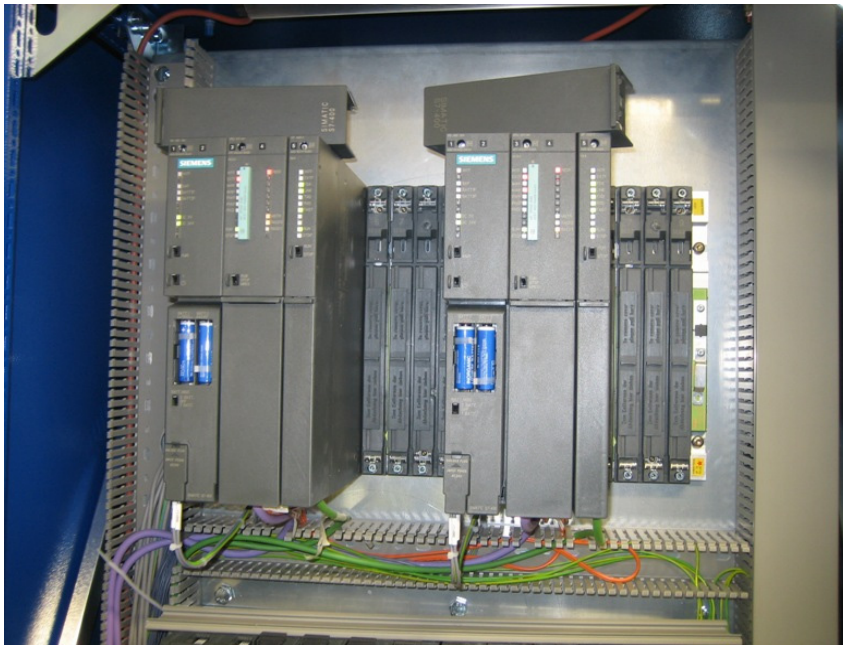
FIGURE 15: Redundant programmable logic controller, PLC
