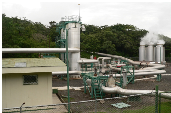
FIGURE 1: Separation station in Miravalles
