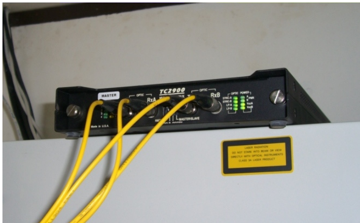
FIGURE 8: The fibre optic multiplexer used in Miravalles
