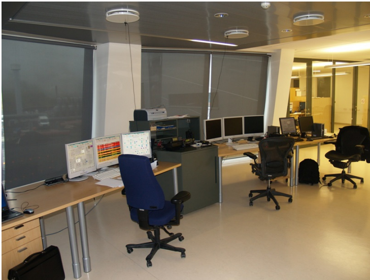
FIGURE 13: Operator consoles in the SCADA control room of Hellisheidi power plant in Iceland
