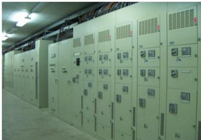
FIGURE 12: Motor control centres (MCC) at Olkaria II power plant
