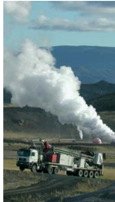
FIGURE 30: View of the trailer mounted Drilmec HH-300 rig
