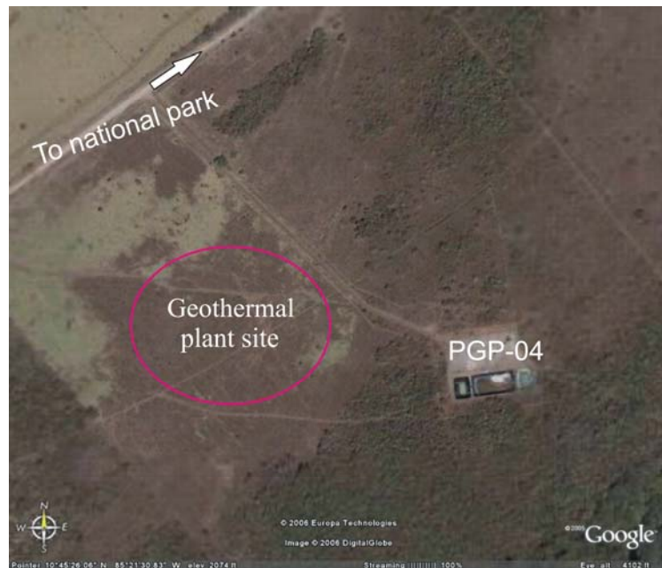
FIGURE 6: Future geothermal plant site and the platform for well PGP-04, in relation to the national park entrance road
