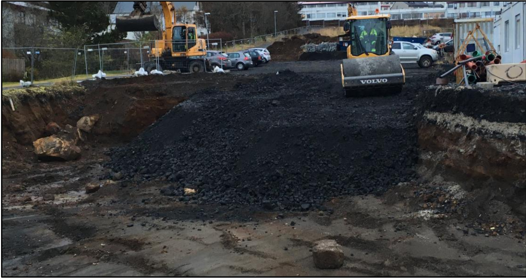
Figure 4. Installation of compacted gravel fill from a profile view at Lundur Site 1 in Kópavogur. The vibro-roller compaction method is shown atop gravel fill underlain by a dense to very dense silty sand base layer.
