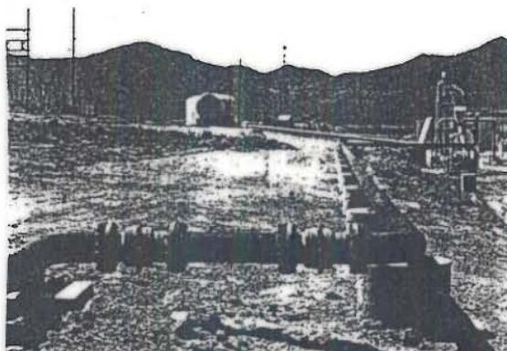
Figure 9. Ball-joint expansion device on pipe line.
