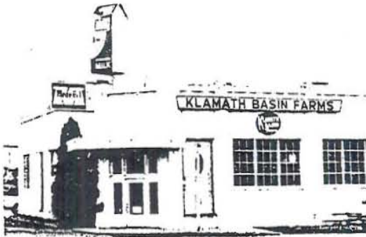
Figure 13. Medo-Bel Creamery with well house and supply line in the left background.
