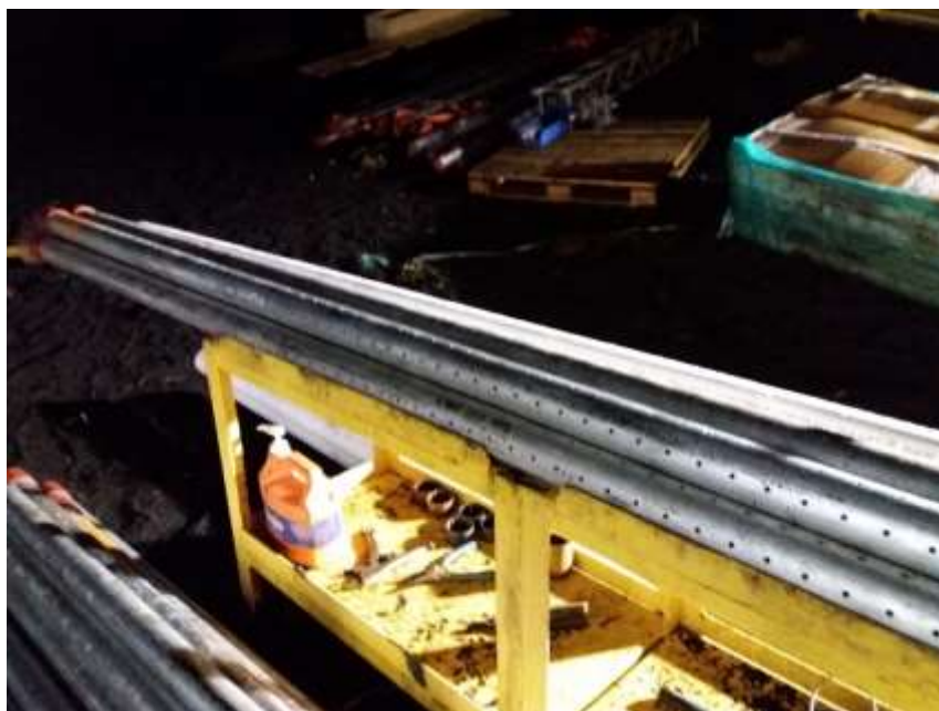
Figure 3. Picture showing slotted Al casing for SE-2b (image TBW).
