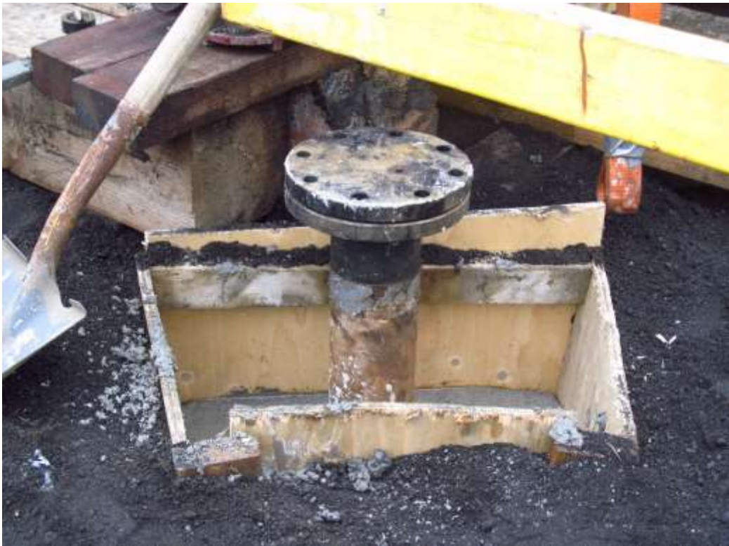
Figure 5. Well-head of SE-2b (image TBW).
