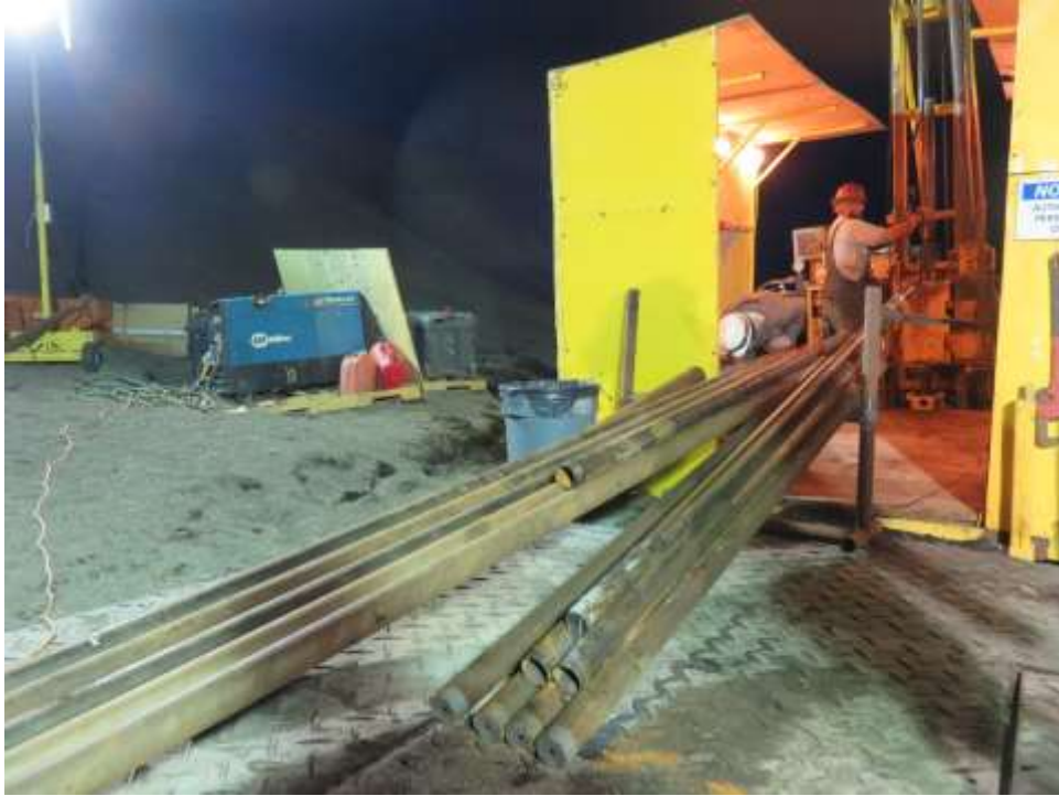
Figure 2. Picture showing the drill rig while coring at SE-2b on Surtsey on August 20 th , 2017 (image source: AB).
