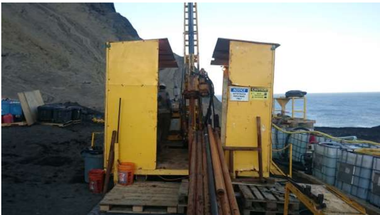
Figure 2. Drill rig with tilted mast (image MTG).
