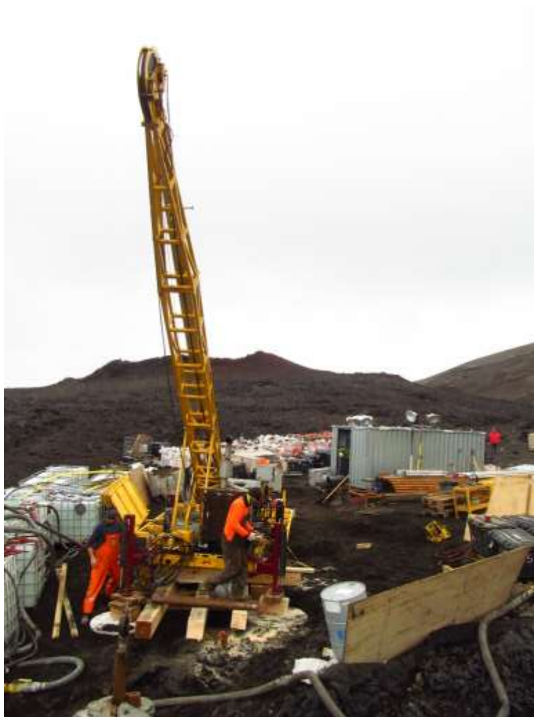
Figure 7. Rig orientated for drilling the angled well SE-3 (image TBW).
