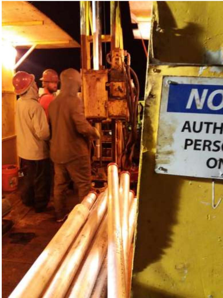
Figure 2. Drilling crew while RIH with the Al casing SE-2b (image TBW).
