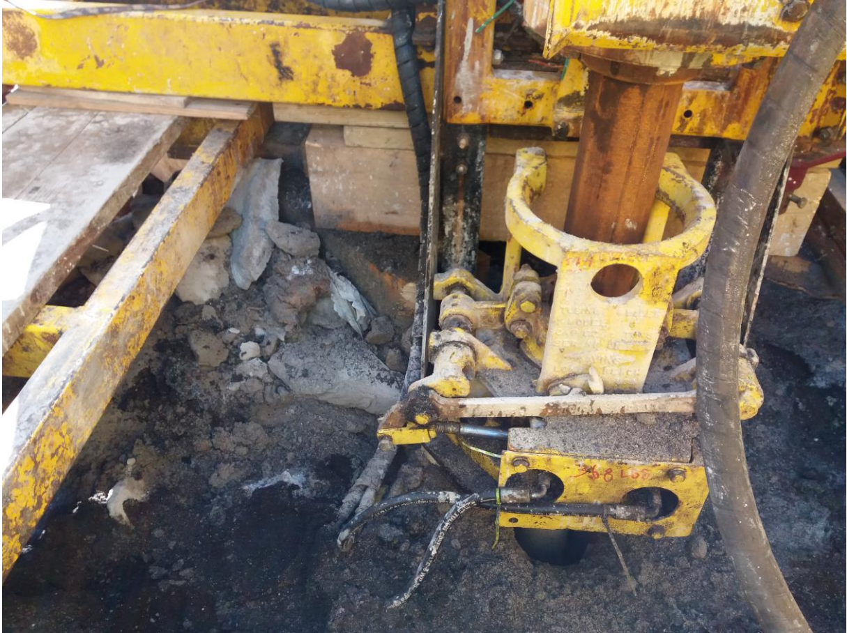
Figure 3. Picture showing cement fragments (left side) that hardened during storage and were not usable for cementing the surface casing of SE-2b (image source: TBW).
