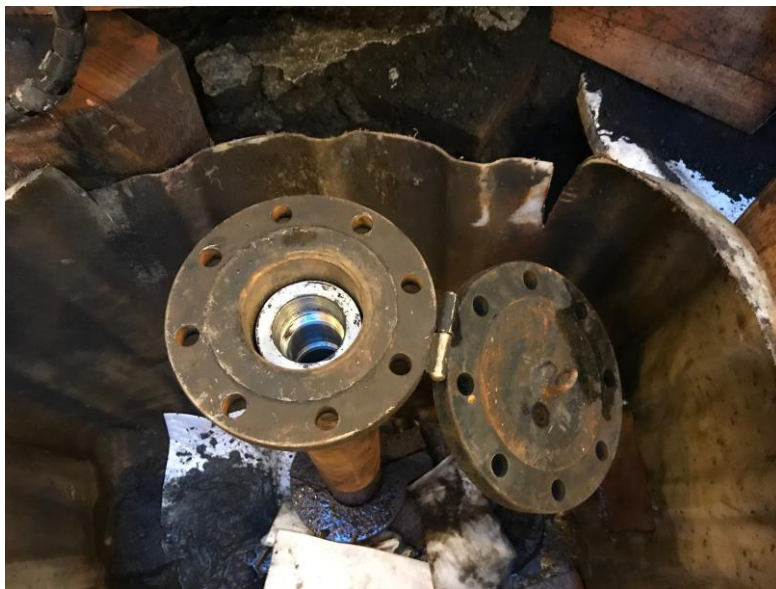
Figure 29. Photograph of the well-head of borehole SE-02b (photo: BM).
