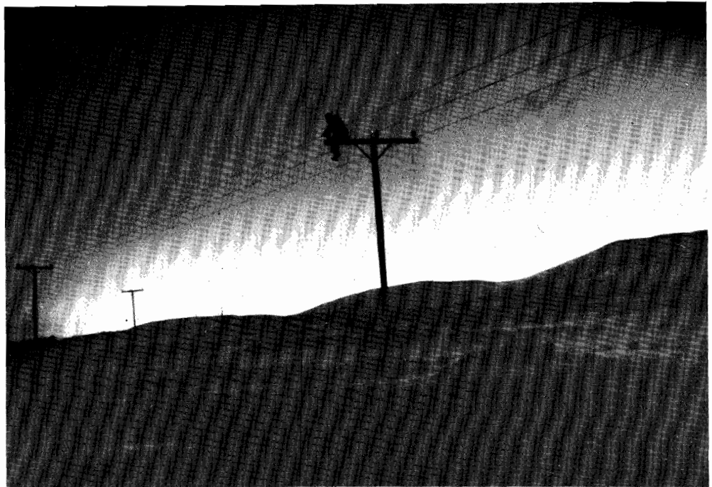
Fig. 4: Electric transmission lines across the rifting zone in Bjarnarflag, south of Krafla. The wires are strained almost to breaking point. The photograph shows a man lengthening the wires in the evening of April 29, during rifting.
