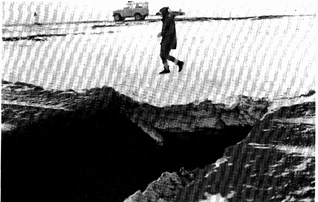
Fig. 6: One of the trenches formed in the Axarfjörður main road. The hardened snow forms a bridge across the trench. See text for explanations.
