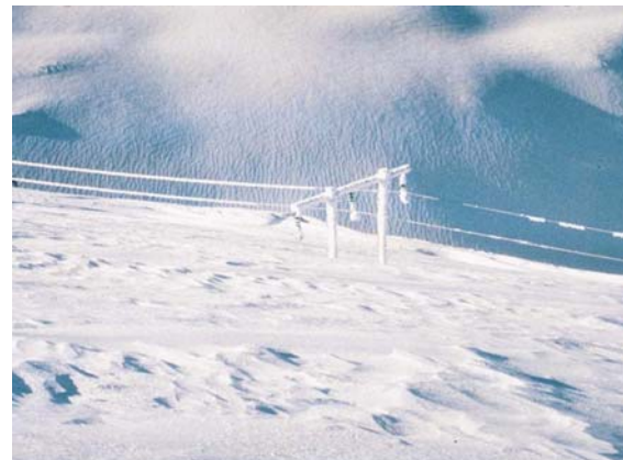
Fig. 9: Severe accumulation of snow.
