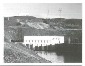
THE SULTARTANGI DAM: The dam, which is 6100 m long, was built in 1982-1983 for a maximum water level at 297 m a.s.l. and a regulated storage of 50 GL. Besides regulating the water flow, the dam reduces the ice formation in the Thjórsá river and the need for flushing of ice past the Búrfell power station. The result is increased capacity in power production. The Sultartangi dam will later be a part of a hydro power station at the Sandafell hill.
